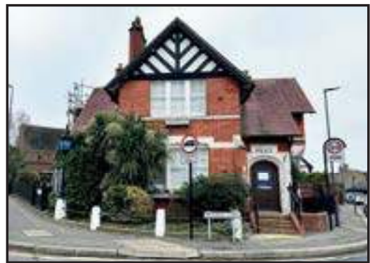
Police Station today
