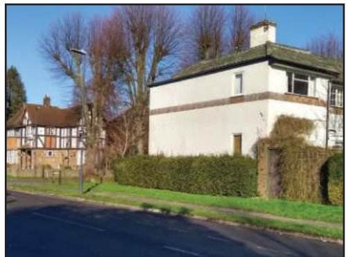
Telecom mast site in North Way
