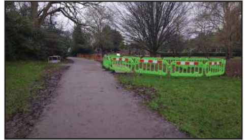
Work in Progress
